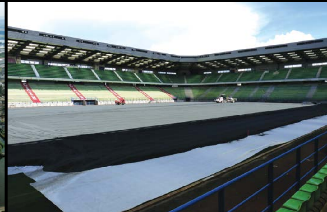
Construction work on D'Ornano Stadium, photo by CO. Normandie 2014
